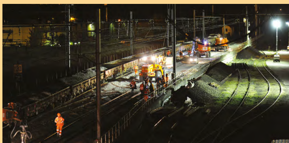
Re-laying track and ballast ©P. Montigny
