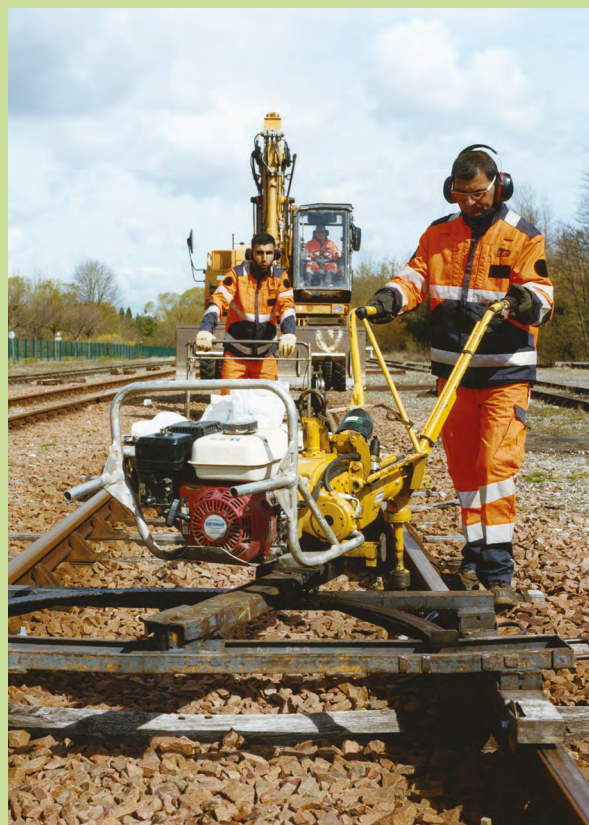
An engineer uses a coachscrewing machine to re-lay sleepers ©Ronan Guillou
