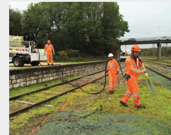
Seeding rail sidings with a hydromulch slurry at Brevans in October 2019 © Anne Petit
