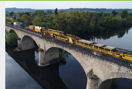
Our track-renewal train in action on a viaduct between Libourne and Bergerac, in south-western France © SNCF
