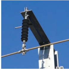
Suspended negative feeder
