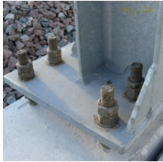
Mast with bolted support
