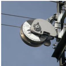
Spring-operated tensioning device
