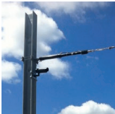
Gas-operated tensioning device
