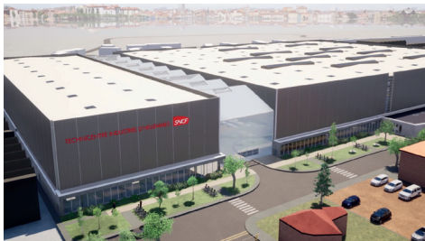
HELLEMMES MAINTENANCE DEPOT IN NORTHERN FRANCE
