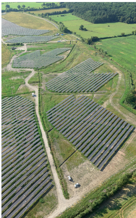
SOLAR FARM OPERATING AT SURDON IN NORMANDY
